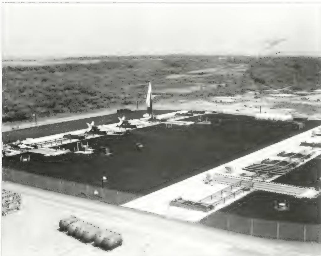
Figure 5.96. View looking northwest at the missile magazines, NIKE launch site, circa 1958. The inner fence surrounding the magazines completely lacked any trace of vegetation when the NIKE facility was operational (GATE 8067).
